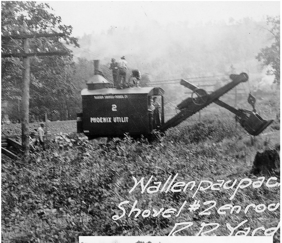
This steam shovel belonged to the Phoenix Utility Co., the builder of the Wallenpaupack project and the forerunner of PPL's Construction Department.
