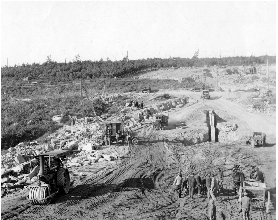
Mules and steam engines provided much of the brawn needed to build the Wallenpaupack dam, as seen in this view of the earthen north embankment of the dam.
