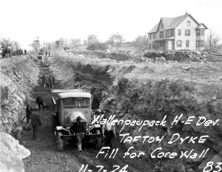
There's more to Wallenpaupack than meets the eye. This 1924 photo shows excavation for the impervious earth fill that has kept the Tafton Dike intact for more than nine decades.
