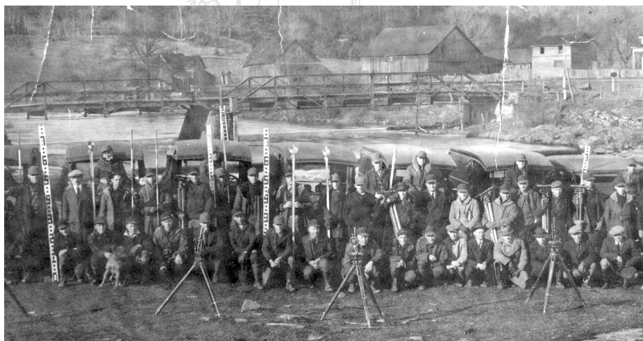
The bridge in the background spans the Wallenpaupack Creek in this 1922 picture showing the corps of surveyors and engineers who were to design Pennsylvania's largest man-made lake.
